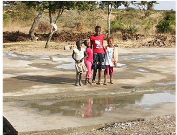
Elizabeth, Amina, Sengenoi and Faith Mumbi on the slab of our new office and two staff quarters.
